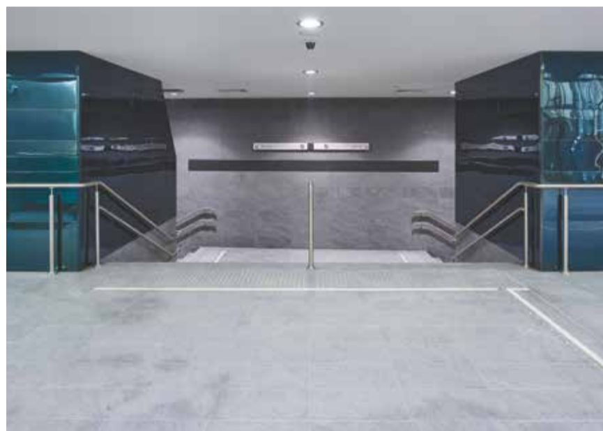
Architectural design: CREW Workshop - Interior design: Studio AEGIS - Team Brescia Mobilità - Photo: Beppe Raso
